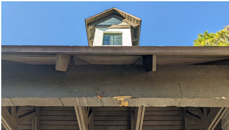
Photograph No.6 – Minor surface damage at the exit of the ranger station
