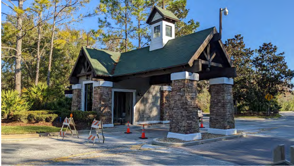
Photograph No.1 –View of Ranger Station
