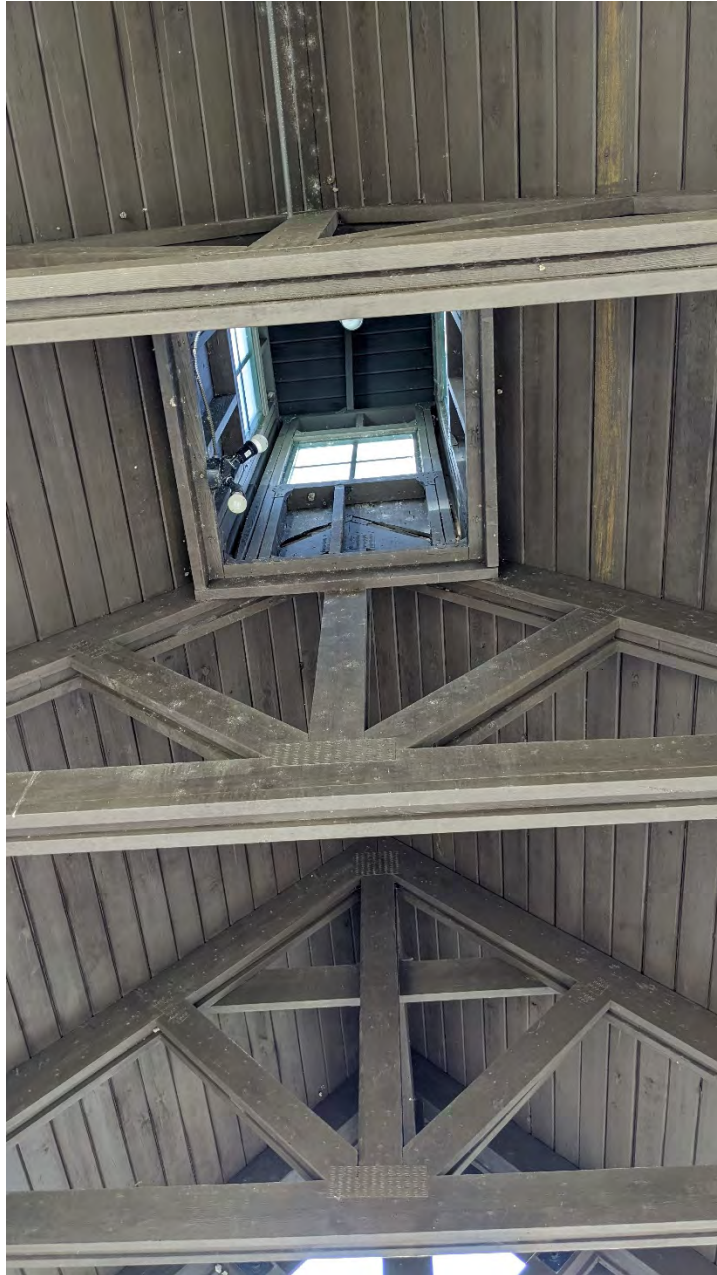
Photograph No.9 – View of wood trusses
