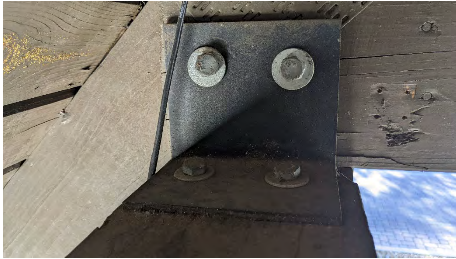
Photograph No.7 – Typical truss tie-down
