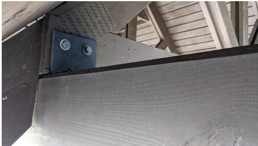
Photograph No.8 – Typical truss tie-down
